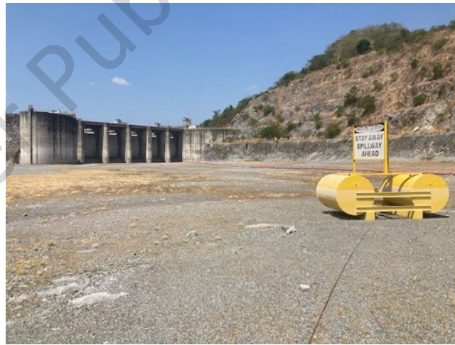
Photo 23: Spillway approach with warning sign
