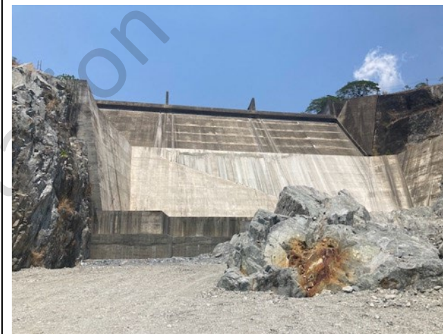
Photo 27: Spillway from below, with additional apron built 2019 to protect from erosion
