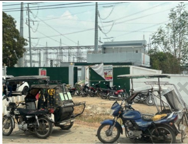
Photo 86: NGCP San Manuel sub-station, south of San Roque
