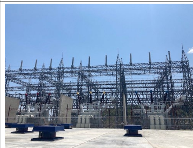
Photo 30: Switchyard and powerhouse roof
