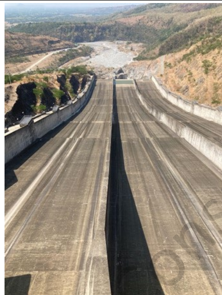
Photo 26: Spillway chutes with aeration lips and skijump at end, powerhouse around river bend to left, floodplain in distance
