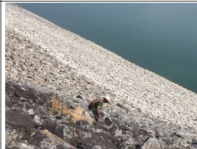
Photo 18: Community worker clearing vegetation from upstream dam slope
