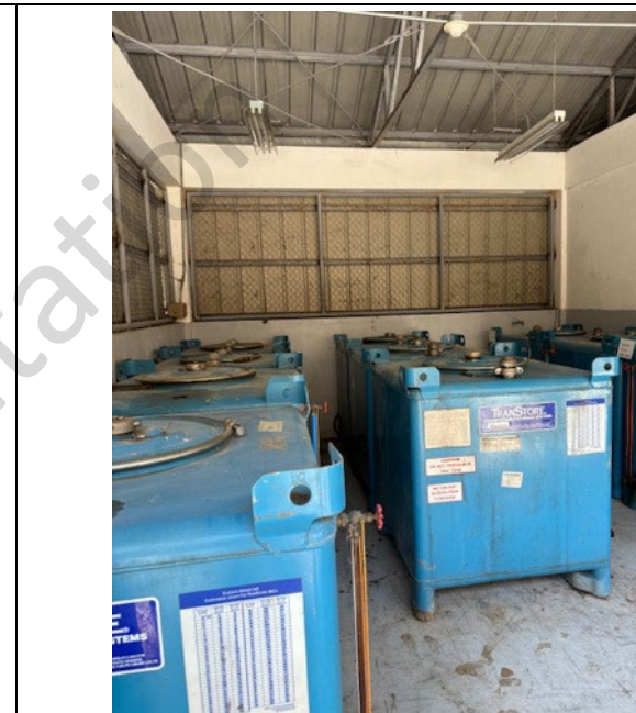
Photo 45: Used oil storage
