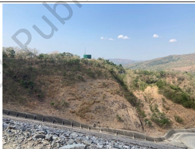
Photo 29: View from dam to surge shaft, showing drainage and protected forest
