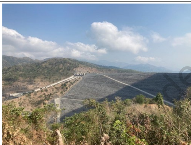
Photo 28: Dam with spillway as seen from surge shaft
