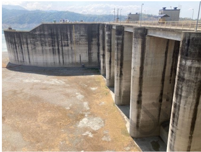
Photo 22: Spillway gates from upstream 2
