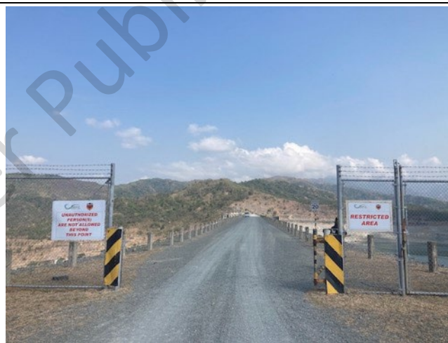
Photo 17: Road over dam crest
