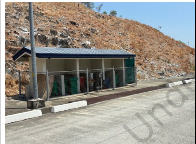
Photo 52: Waste separation near switchyard
