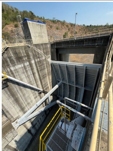
Photo 25: Spillway gate from downstream
