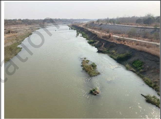
Photo 87: Agno River downstream in floodplain, with embankments
