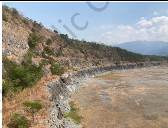
Photo 11: Excavated benches upstream of spillway, with material used for dam rockfill
