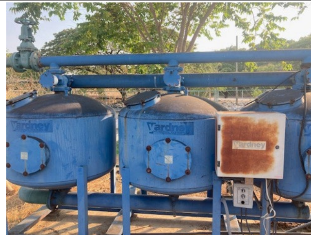
Larawan 54: Water filtration para sa operator's village
